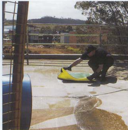
Stormwater Drain Seal
